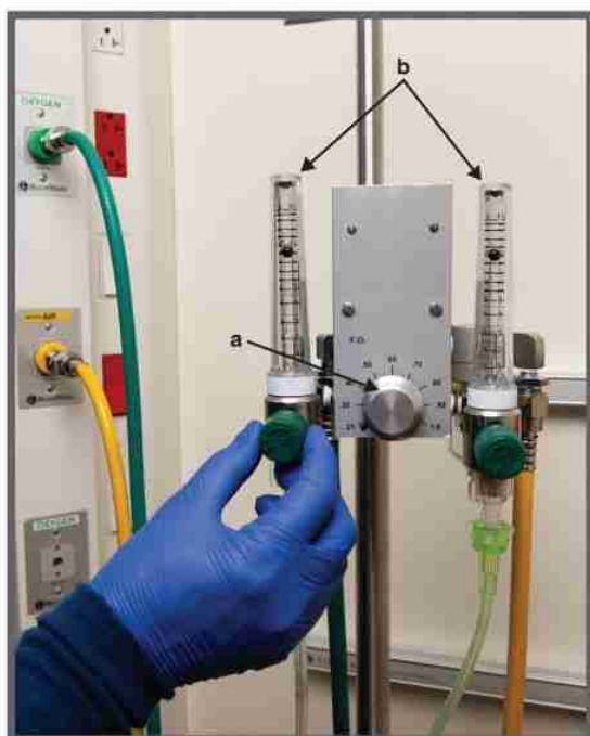
Figure 3.16. Adjust the concentration and flow of oxygen with compressed air (inflow from yellow hose), compressed oxygen (inflow from green hose), an oxygen blender (a), and a flowmeter (b). The blender adjusts the concentration of oxygen, and the flowmeter adjusts the flow of gas. This image shows 2 flowmeters attached to the oxygen blender. Your system may only have a single flowmeter.
